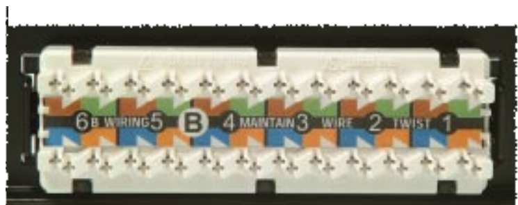
Figure 4: Closeup of the rear of a 6-port module showing the label and wiring configuration
